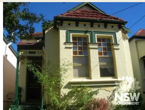
Figure 7.16 Primary elevation of 37 Wallace Street, Burwood, July 2020. (Source: NSW SHI)
