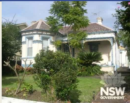
Figure 7.3 Primary elevation of 12 Belgrave Street, Burwood, July 2020. (Source: NSW SHI)
