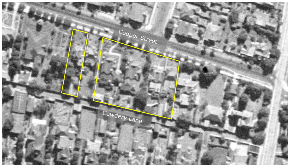
Figure 5.4 A 1943 aerial photograph of Cooper Street showing the subjects sites outlined in yellow. (Source: NSW Spatial Services)
