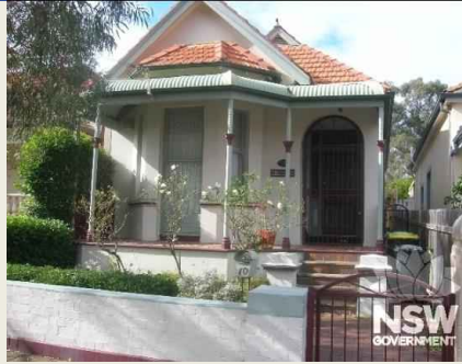
Figure 7.5 Primary elevation of 12 Bold Street, Burwood, July 2020. (Source: NSW SHI)
