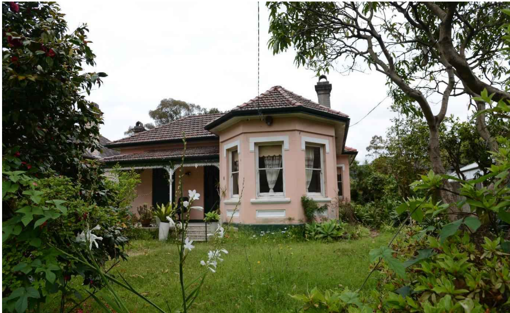
Figure 6.8 Northern façade of 6 Cooper Street, viewed from Cooper Street.
