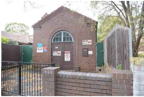
Figure 6.3 Heritage listed substation at 2B Cooper Street.
