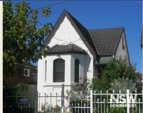
Figure 7.8 Primary elevation of 2A Brooklyn Street, Burwood, July 2020. (Source: NSW SHI)
