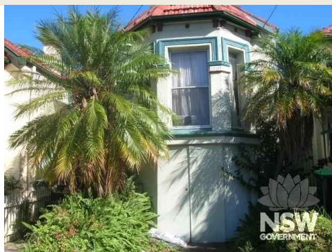
Figure 7.15 Primary elevation of 35 Wallace Street, Burwood, July 2020. (Source: NSW SHI)
